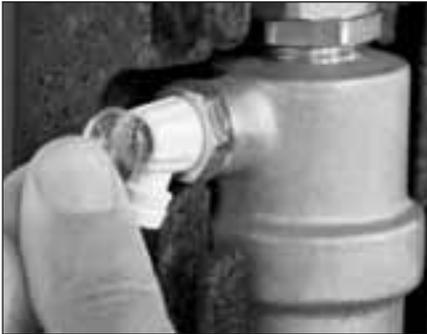
2) *Manually open air vent located in pumping station. Air should also expel from here. When fluid begins to expel, close vent.*
