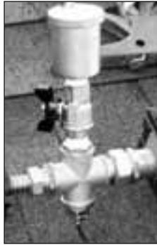
1) *If it is used, open up the air vent ball valve on solar panel. You will likely hear air being expelled from air vent.*
