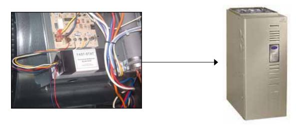
2. The Sending Unit is connected to the existing thermostat cable and the new thermostat. The Sending Unit is then installed into the wall space behind the thermostat
