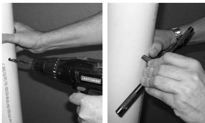
Figure 9.1: Drill and Tap Combustion Test Port
