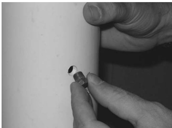
Figure 9.3: Insert Pipe Plug into Test Port
