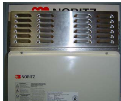
Figure 3b: Vent cap installed.
