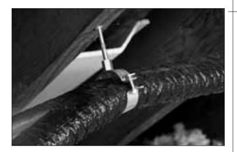
• Any piping through the attic or basement should be properly supported. We recommend supporting Solar Flex every 36 inches. A hanger kit of 4 brackets is included in the parts box.
