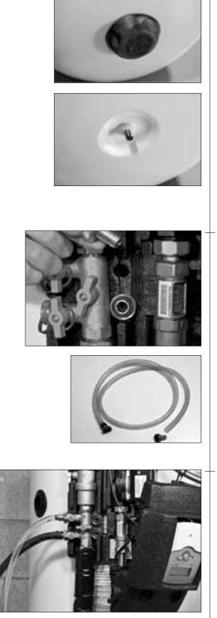
• Adjust expansion tank pressure to equal the solar loop pressure. Black cap spins off revealing valve.
