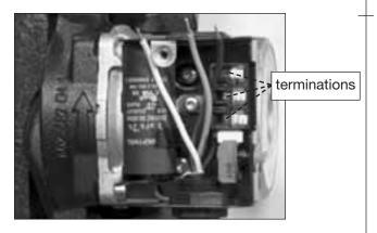
• Unscrew plate from front of pump. Run 18 inch "J cord" that comes with kit up through the bottom strain relief port. Connect the 3 wires into the motor. Consult the included Pumping Station installation instructions for more details on wiring motor.
