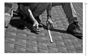
For each panel, choose the best intersections to place 2 mounting brackets and ensure good panel support. Bracket locations should be no more than approximately 12" away from the panel side.
