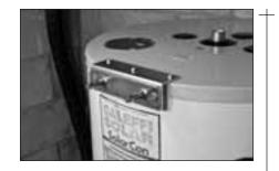
• Place the angle bracket on top of storage tank where you want to mount the pumping station. This is usually directly above the heat exchanger ports to simplify piping. Drill 3 shallow pilot holes, and then use the supplied self tapping screws to mount the bracket assembly to the tank.
