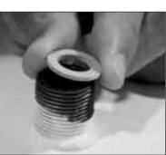
• Connect the expansion tank hose ends to the pumping station and check. Remember to use washers.
