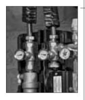
With the pump station mounted onto the wall or solar storage tank, cut to length and install the Solar Flex coming from the roof onto the top connections.
