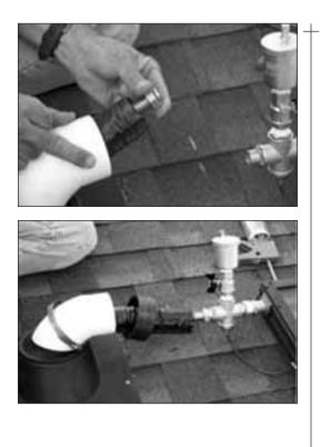
• With the Solar Flex union now assembled, connect to the cross.
