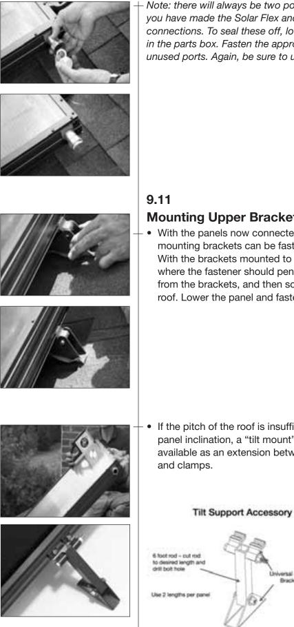
Note: there will always be two ports left unused once you have made the Solar Flex and cross assembly connections. To seal these off, locate the plugs or caps in the parts box. Fasten the appropriate fitting into the unused ports. Again, be sure to use a green washer.
