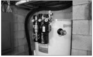
The pump station components can now be re-assembled to the bracket. First install the rear foam cover over the brackets. Then push the two pump station assemblies onto their respective pins on the mounting bracket. A click sound will indicate the components are locked securely onto the pins.
