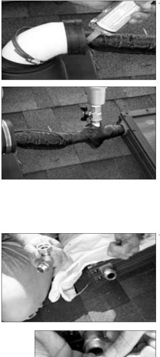
• Put Fernco cap in place. Seal off using any remaining openings with roof cement. Tighten up clamp. Run the panel sensor wire down through roof. A helper can simplify this task.
