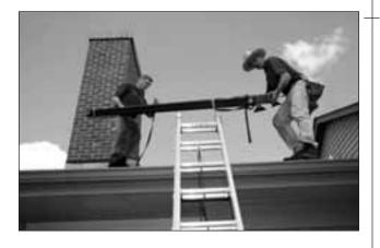
• Web (or rope) lifting slings are suggested for lifting panels onto a low single story roof. Using a ladder facilitates lifting. A typical method is two people on a roof pulling ropes while a third person on the ground helps push the panel upwards.
