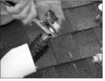
• Have a helper assist in pulling one side of the split Solar Flex up through the hole (or holes) in the roof. Attach the union nut and stainless clip ring using the folowing procedure.
