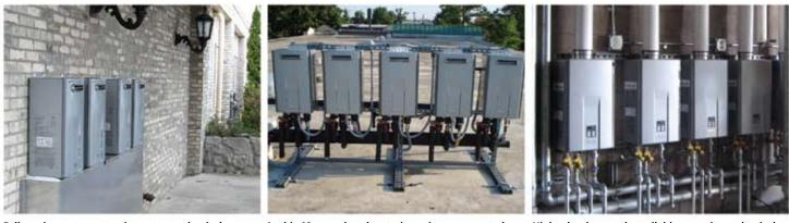
Full service restaurant gains extra mechanical room square footage for additional storage plus redundancy by installing multiple units on the exterior wall.
