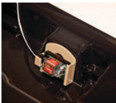
Probe Sensor (Mounted to Side of Unit) Auxiliary Drain Probe (Inside Primary Pan)
