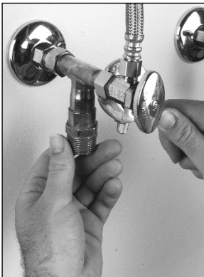
2. Install tees and attach angle stops.
