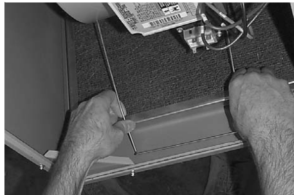
Figure 6 Wire Filter Retainer
